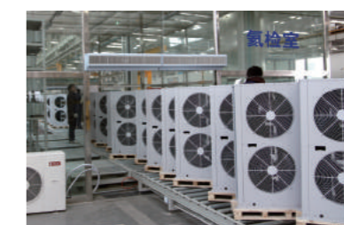
Leak detection systems (Helium)
